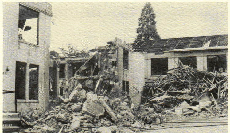
Back view of Hart Hall where recent demolition is most evident.
