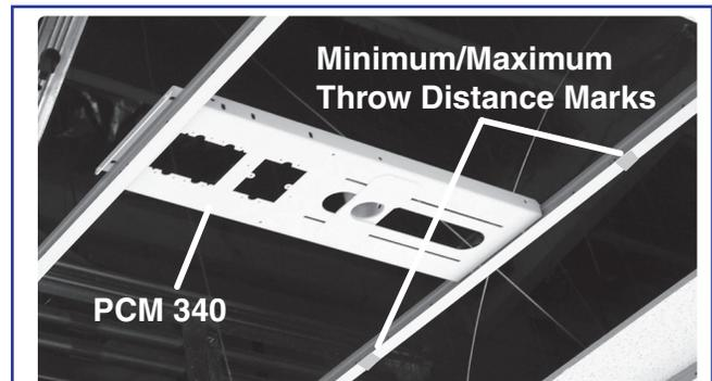
**2b** Place the PCM 340 on the T-bar.
