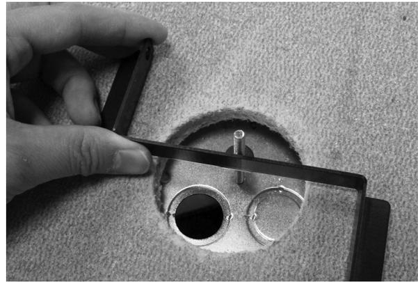
**2 Attach the Z bracket to the ceiling tile and the back plate.**
