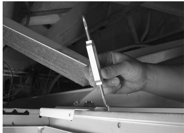
**7a** Attach the turnbuckles at the corners of the PCM 340.
