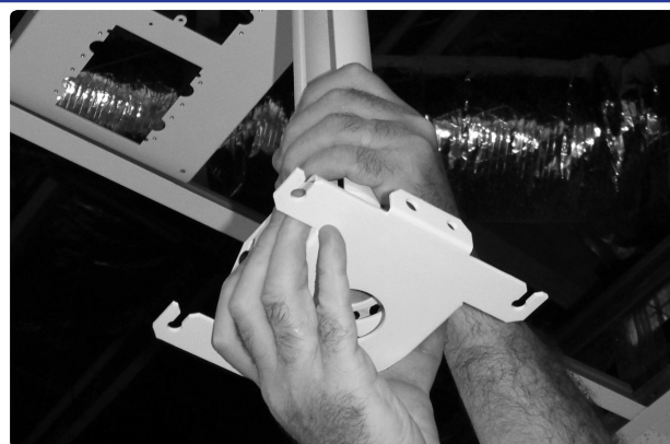
②③ Screw the adjuster plate onto the base of the pipe.
