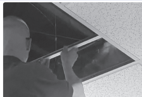
2a Place the T-rails on the T-frame.
