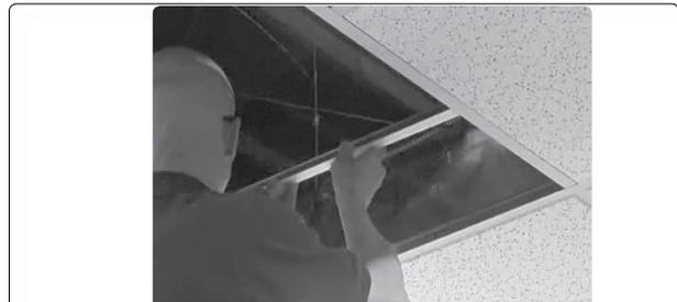
**2a) Place the T-rails on the T-frame**
