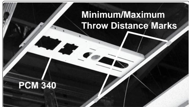
2b Place the PCM 340 on the T-bar
