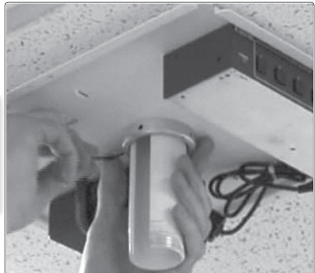
**(2d) Slide the base plate up onto the pole and (2e) secure with the set screws**
