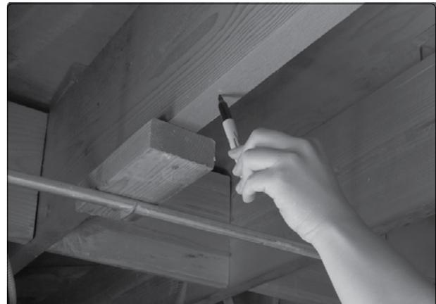
**5a** Mark structural ceiling for lag eye bolt installation
