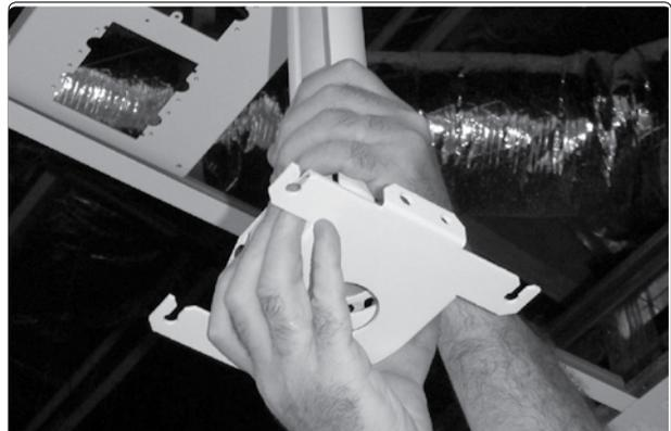
2d Screw the adjuster plate onto the base of the pipe.
