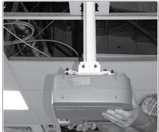
**2f** *Slide and lock the projector onto the adjuster plate*
